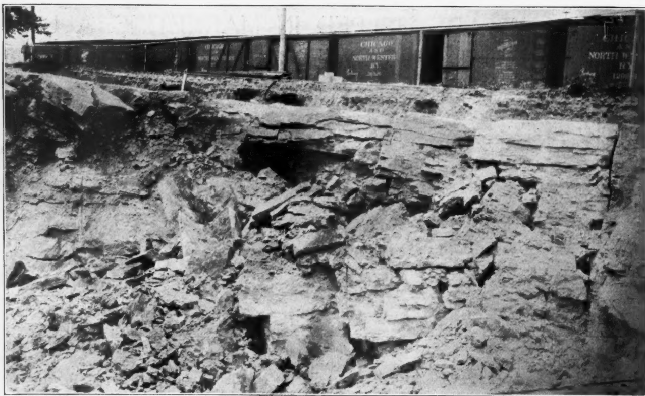
Deposit After Shot Has Been Fired
